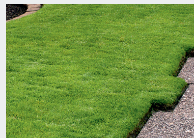
Pavement cleaning and landscaping
