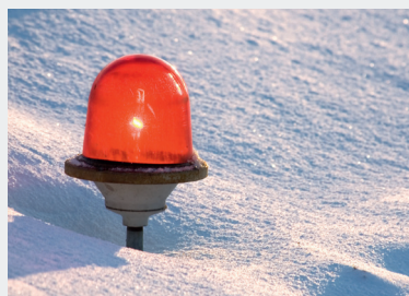
Snow removal at airports
